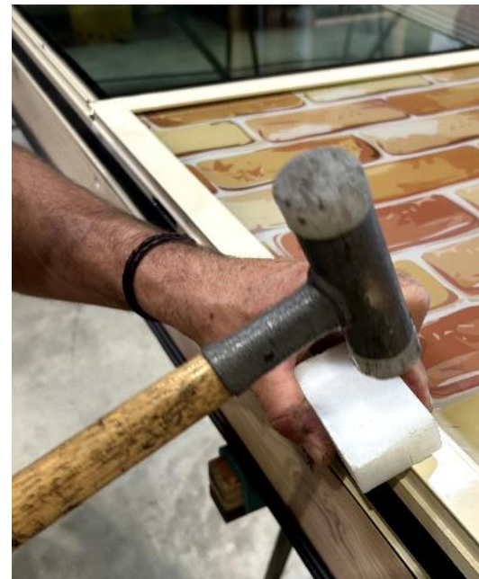
Glazing bead installation
