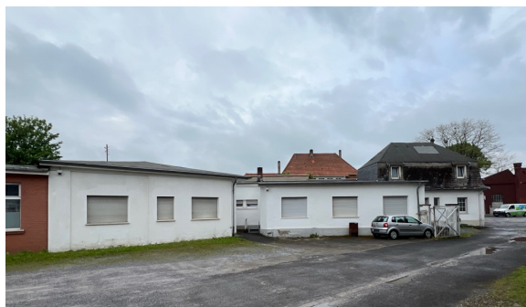
Menden, Germany Refurbishment of an office building now used for housing
