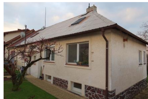
Czech Republic Refurbishment of suburban semi- detached house
