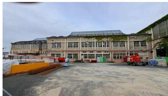
Vitry-sur-Seine, France Refurbishment of former train maintenance into offices
