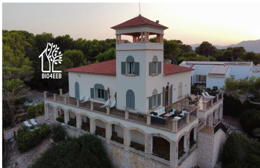
Mallorca, Spain Historical and protected residential complex refurbishment
