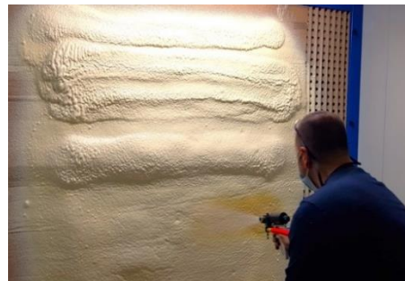
Figure 1. Bio-based PUR formulation spraying
