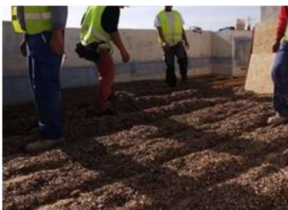
Figure 4 - Insulations from Posidonia Oceanica fibres (Photo Fraunhofer ICT, (left) NeptuTherm (right))
