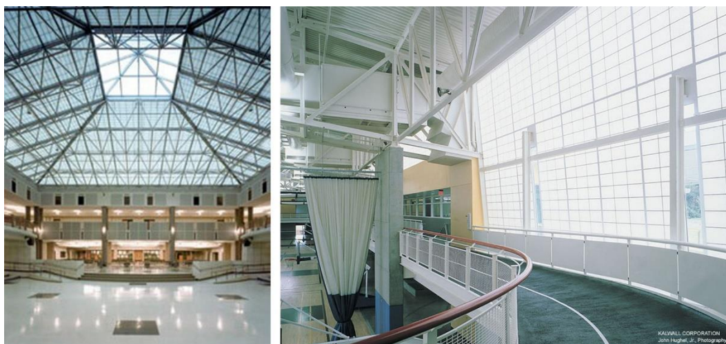
Figure 8- Examples of translucent aerogel insulation as a high performance thermal insulation solution for daylighting (retrieved from Baetens et al., 2011 ).
